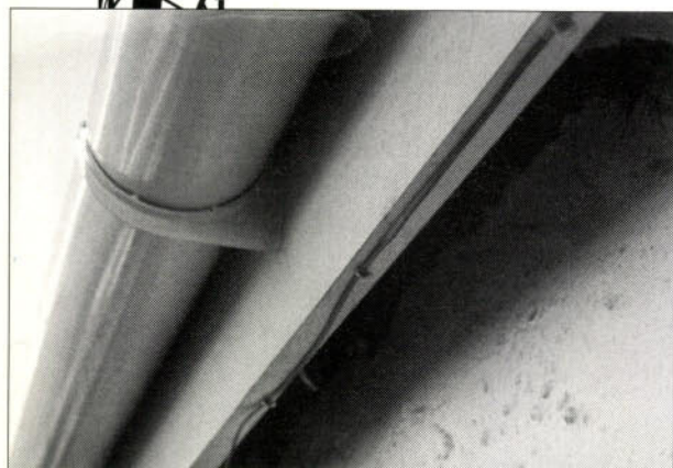
Fig. 2: The wire under the eaves would not be seen at all if it were fitted behind the fascia or behind the soffit board.
