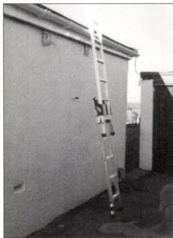
Fig. 5: Stepping up the h.f. band. A metal ladder makes a good vertical antenna if loaded against a counterpoise.
